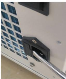
Turn off the device and disconnect the power cord. Lift the fuse holder cover with a flat screwdriver. Remove the fuse and check if any blackout is visible. If there is, replace the fuse immediately.
